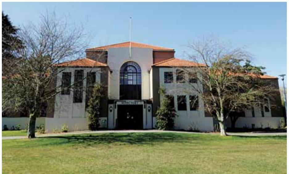
The heritage Refectory building to be restored and refurbished
